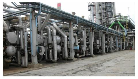
The good heat transfer (clean exchanger surfaces) is important from energy efficiency viewpoint Upstream of the desalter the crude oil is heated up to 130-140 °C
